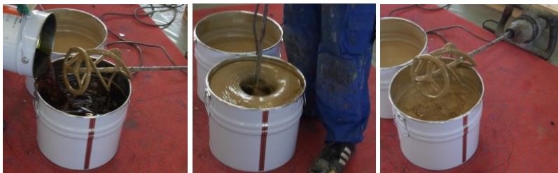
Mixing of the 2-component PU adhesive
