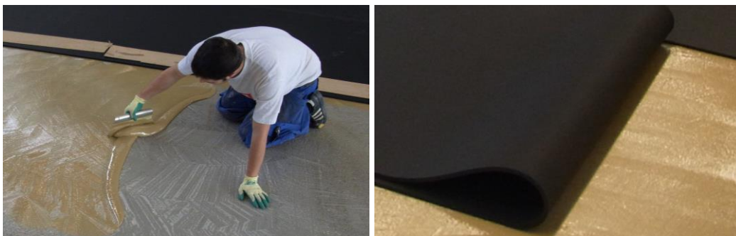
Adhesive applying onto clean substrate; roll out into the adhesive bed
