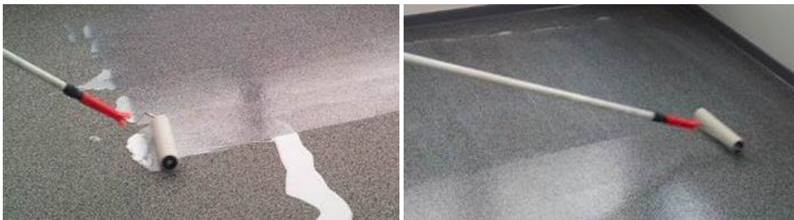
Applying of the coating
