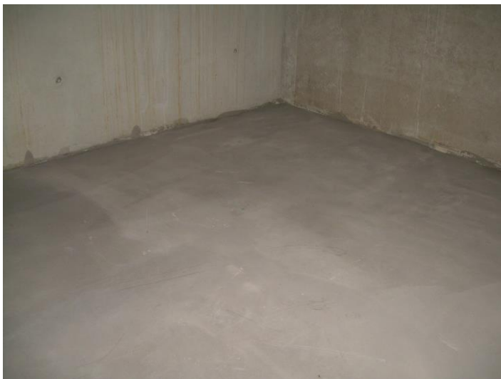
Even, suitable substrate made of poured screed
